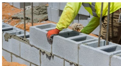
General Masonry Projects
