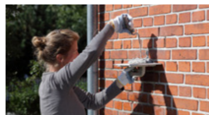
Pointing & Patch Repair Jobs
