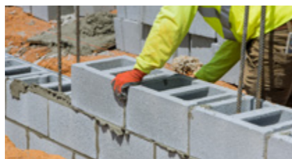
General Masonry Projects
