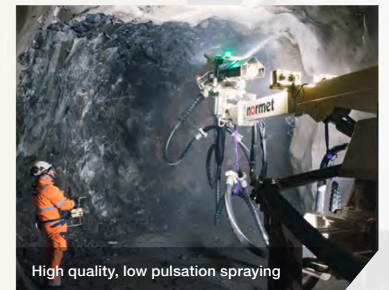
SmartScan Align providing thickness control
