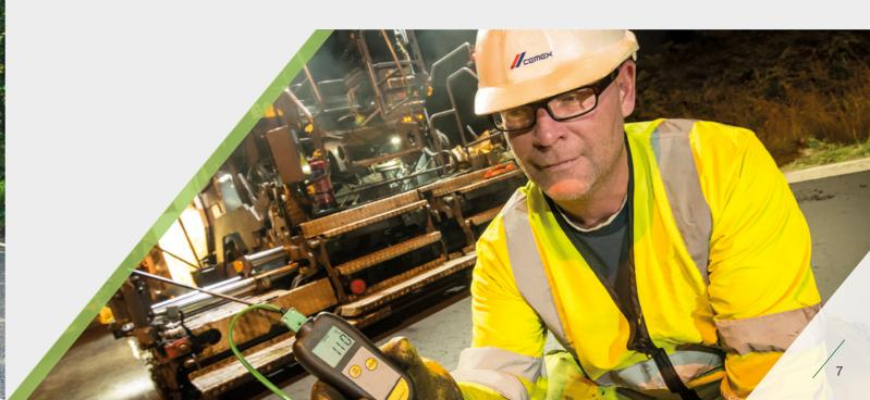
the construction site. The reduced mixing and paving temperatures of low temperature asphalt can cut fume generation by around 50% for approximately each 10°C reduction in temperature.
